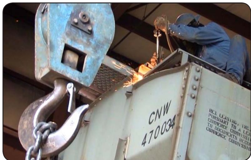
A member of the mechanical services team works to repair the top of a railcar.
